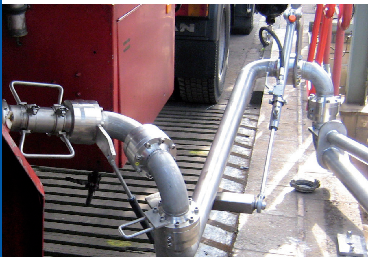
Bottom loading station vapour return arm on top, product arm underneath insulated and electrically heated
