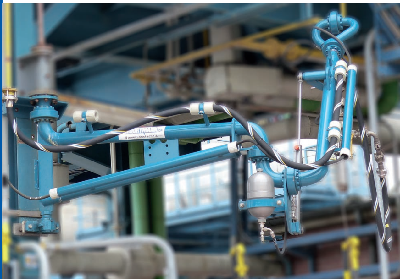
Loading arm with guided nitrogen hose
