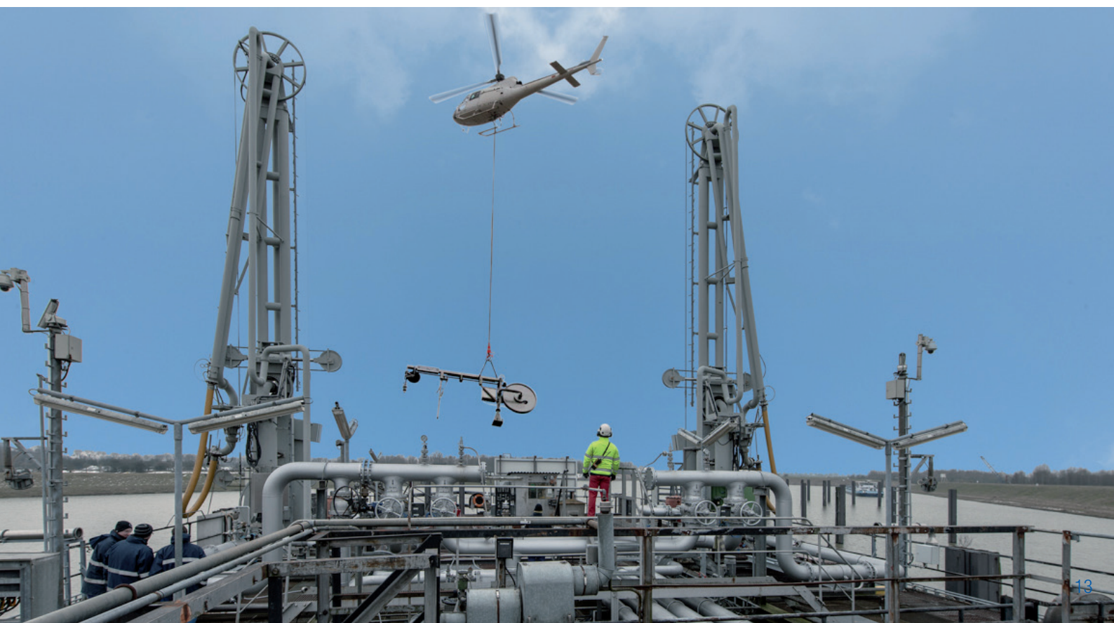
Delivery and assembly of a hose handling system for residue removal
